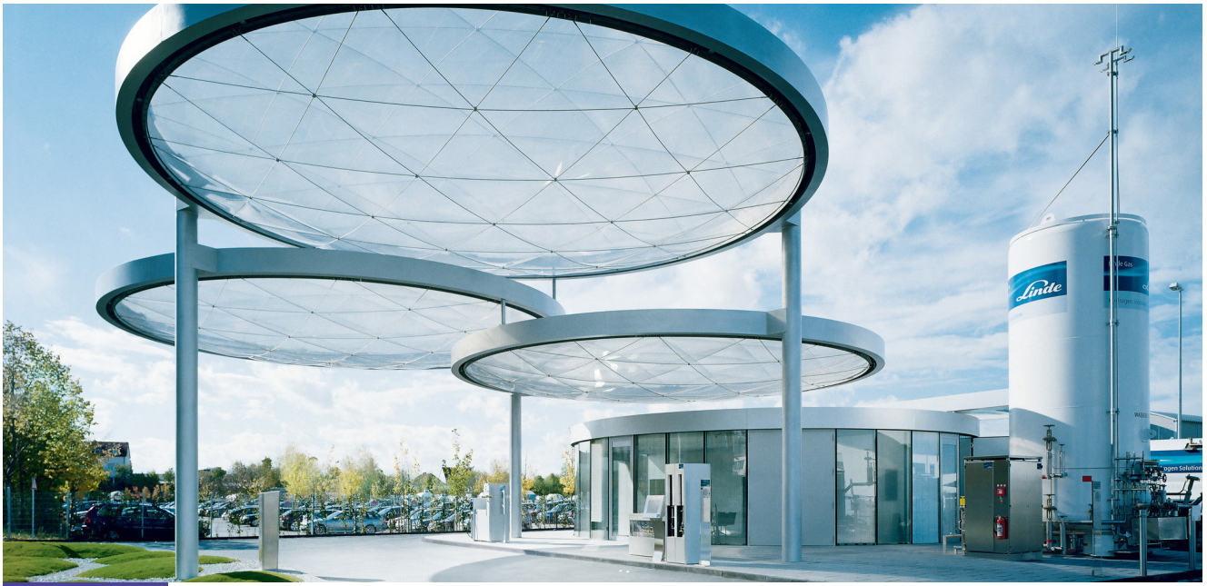
Linde Hydrogen Centre, Unterschleissheim, Germany
